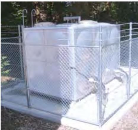
Operation at Okaya City
